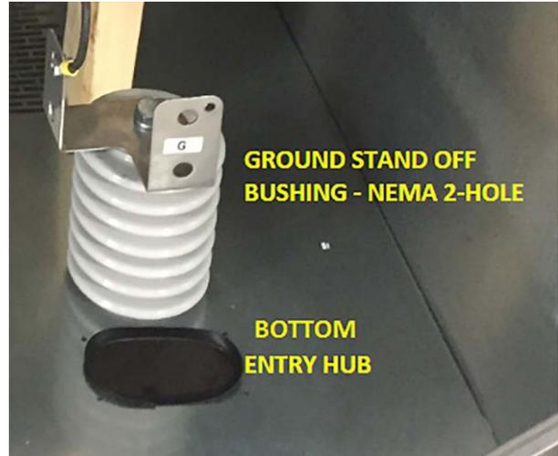
Example of bottom mounted bushing for N/G connection
