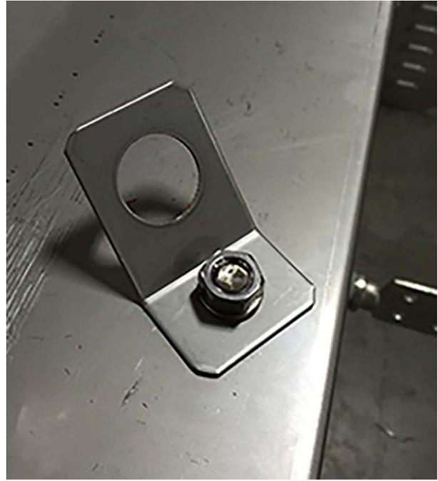
Example of top-mounted lifting eyes
