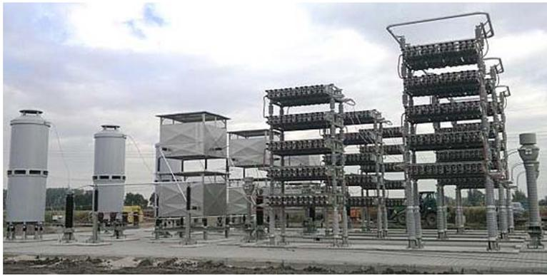
**Figure 3: To master the high voltage of 250 kV to 300 kV phase-to-ground in accordance with the regulations, frames are developed for the capacitors, upon which each horizontal assembly is installed using individual capacitors. These frames are separated electrically using insulators and assembled at the customer site to form a tower 7 m to 10 m high. A total of 30 to 45 frames are required depending on the power of the plant.**
